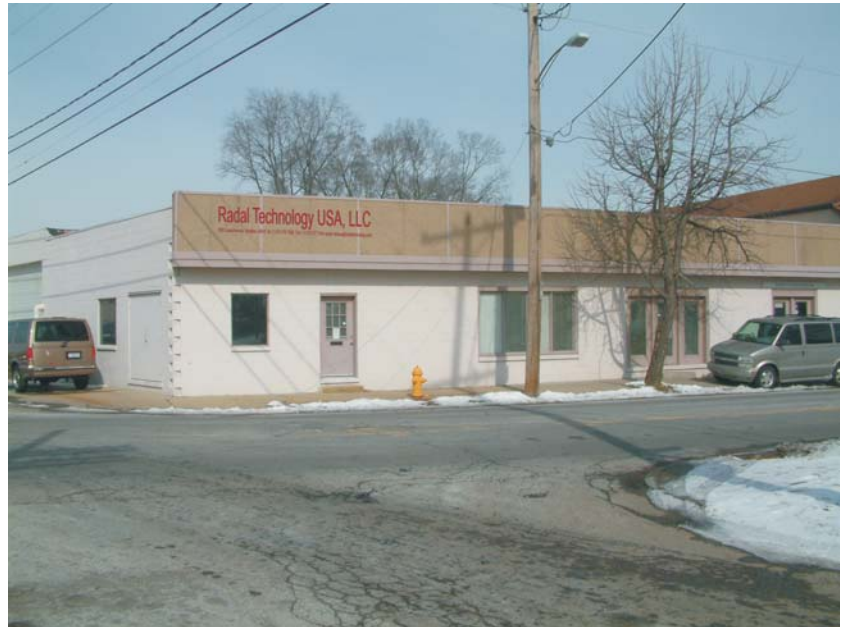
Radal’s new office/warehouse facility based in Hamilton Ohio
